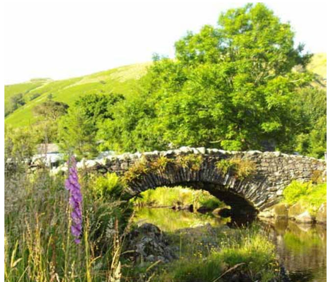
Watendlath packhorse bridge © Caroline Millar
